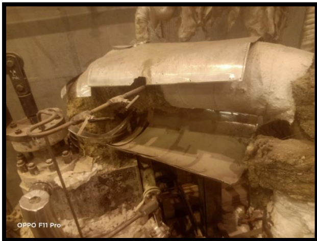
Remove Insulation Refractory
