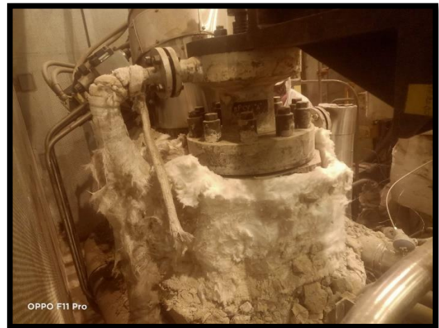
Remove Insulation Refractory
