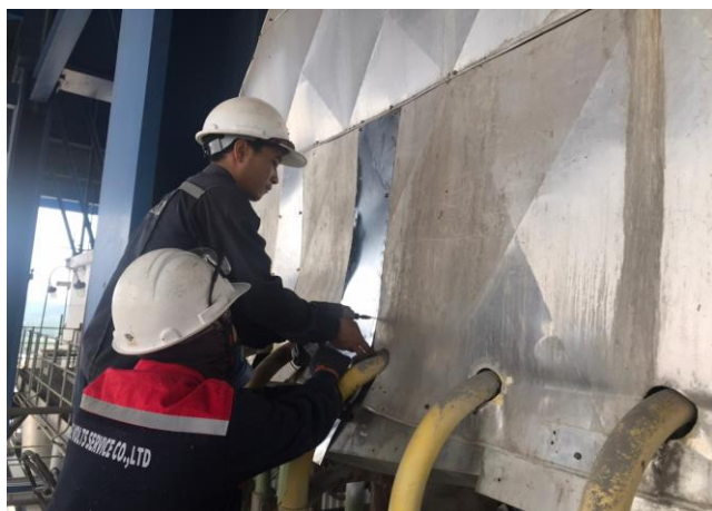
Re-Install Insulation Lagging
