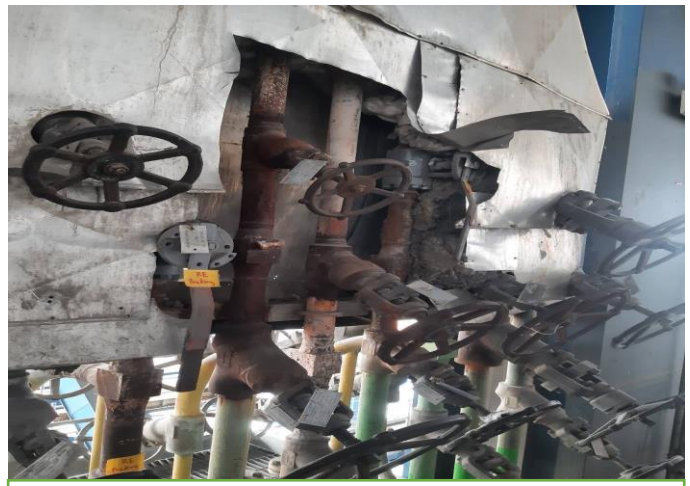
Remove Insulation Lagging
