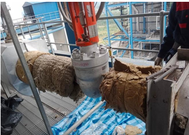
Remove Insulation Lagging
