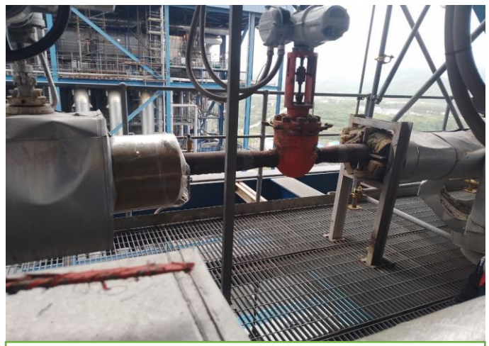
Remove Insulation Lagging
