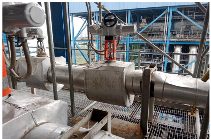
Remove Insulation Lagging
