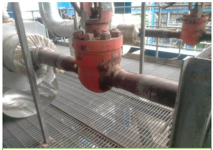
Remove Insulation Lagging
