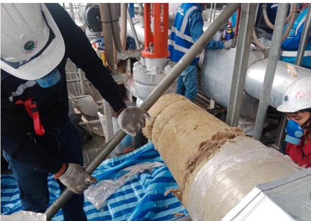
Re-Install Insulation Lagging
