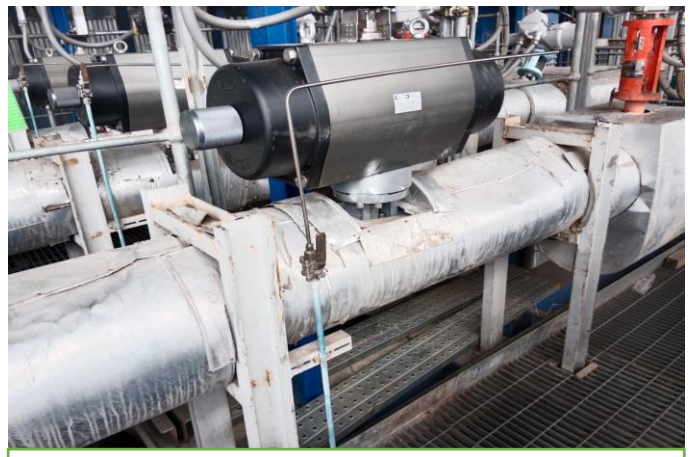
Remove Insulation Lagging
