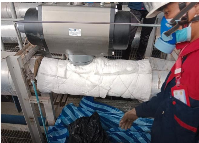
Re-Install Insulation Lagging
