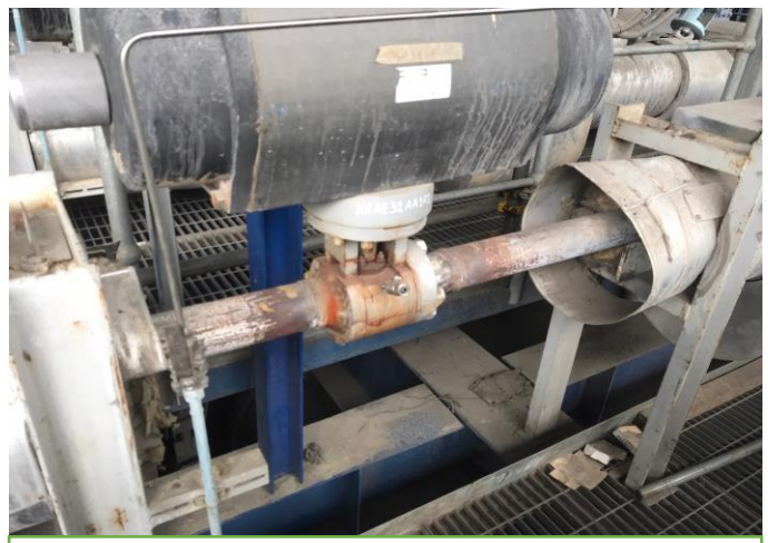
Remove Insulation Lagging
